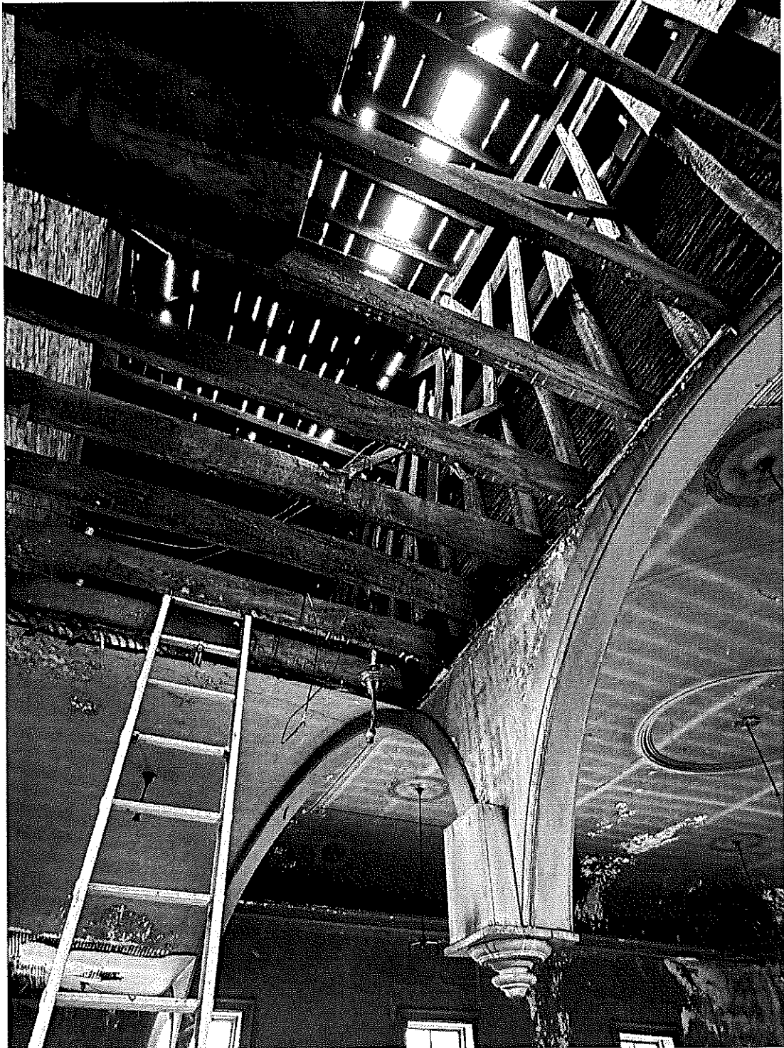
Photo 17 – South Building between South Wall and first roof truss
