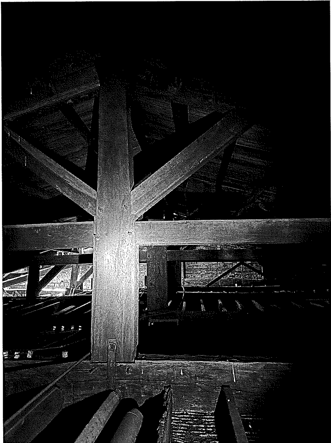
Photo 13 - South Building Truss, center
