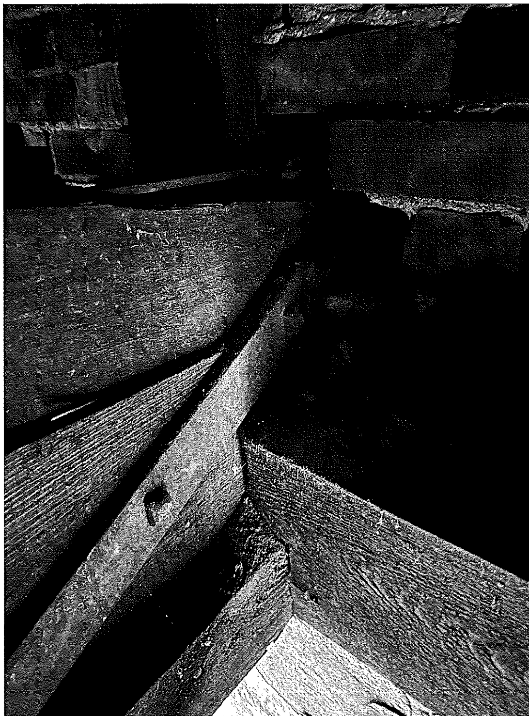
Photo 5 – North Building roof truss bearing at North wall.
