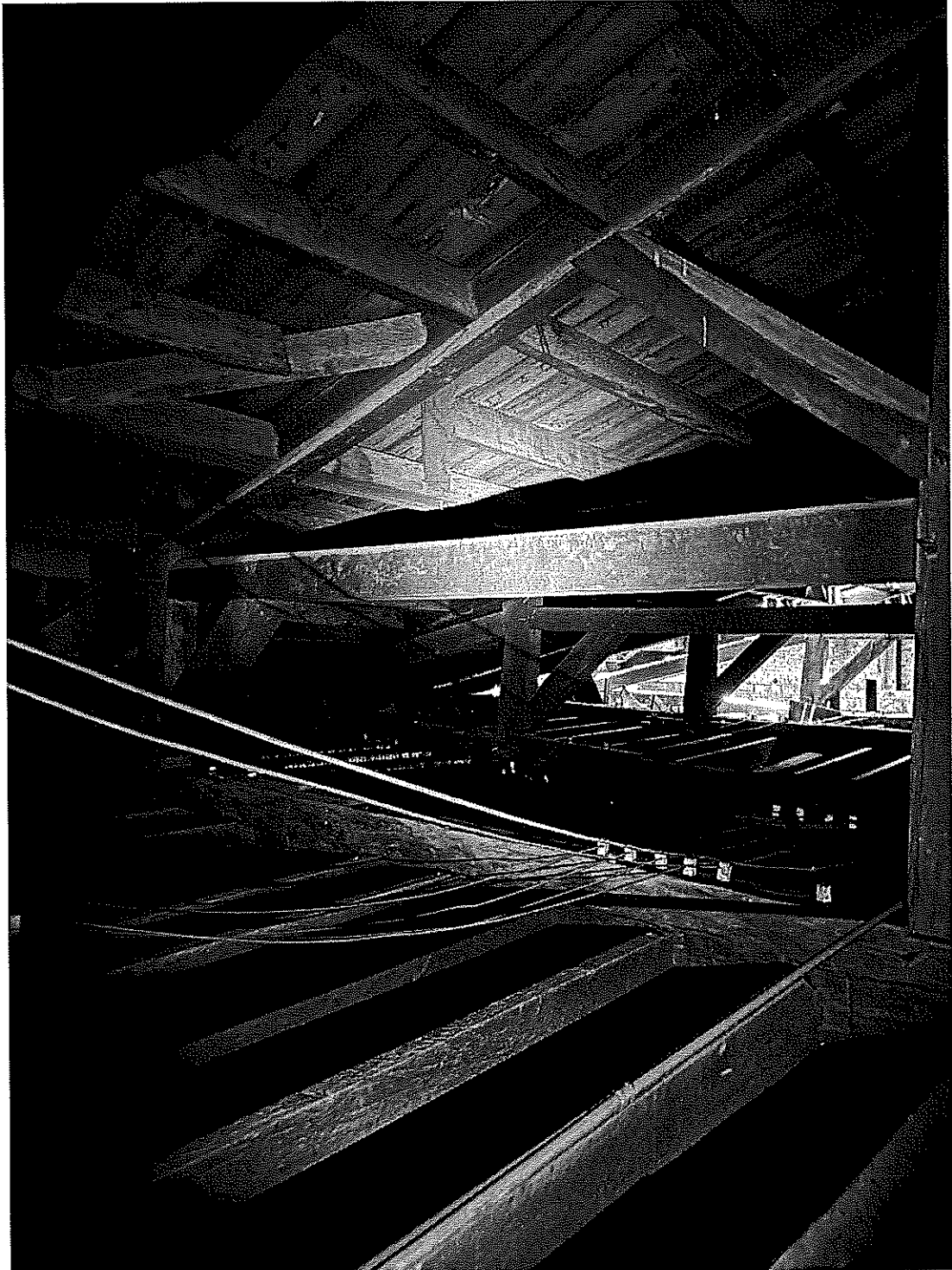
Photo 12- South Building Truss, East half
