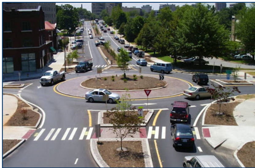
Figure 13: Pedestrian Refuge Islands (Source: FHWA)
