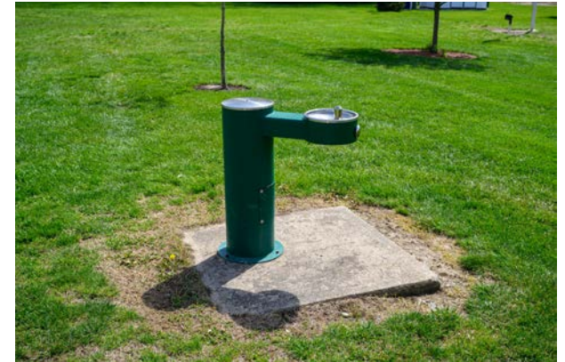
Accessible connection needed to water fountain in Trostel Park.
