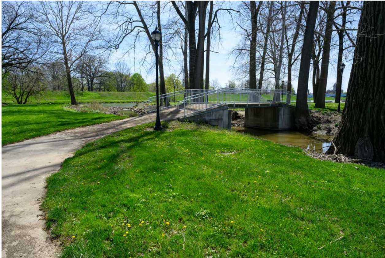
The pedestrian bridge to the central island at Treasure Island may be too steep for some visitors to navigate. Since boats can access the restaurant on the other side of the island, a lower bridge here would increase access for all.
