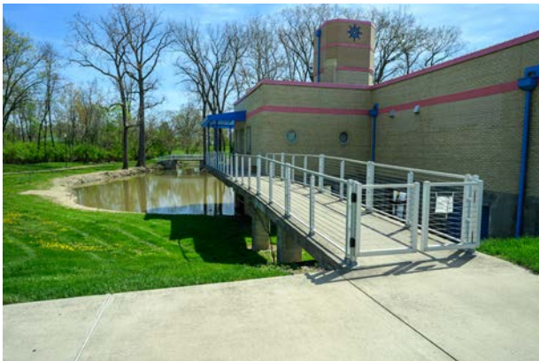
An accessible ramp with railings at Treasure Island Park.
