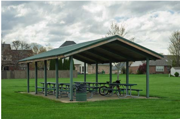
The picnic shelter at Carriage Crossing Park should include at least one ADA-compliant table and be connected to the overall sidewalk/pathway system of the park.
