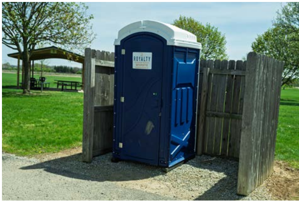
When there is only one porta-potty in an area, like this one at Duke Park, it should be ADA-compliant and have continuous pavement up to its doorway.
