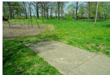
Where sidewalks currently end, such as this one in Community Park, connections should be installed to make the accessible path continuous.
