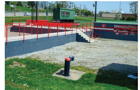
Water fountains at the North Market Ball Fields should be replaced with accessible ones connected to the sidewalk/pathway system.
