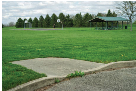
At Carriage Crossing Park, a curb ramp is ready for the rest of the pavement connections to be made within the park.
