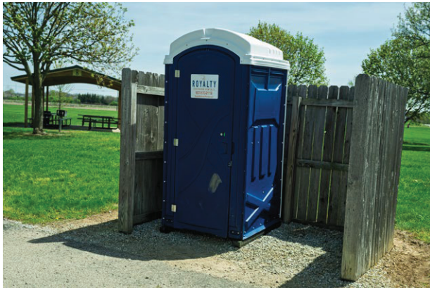
When there is only one porta-potty in an area, like this one at Duke Park, it should be ADA-compliant and have continuous pavement up to its doorway.
