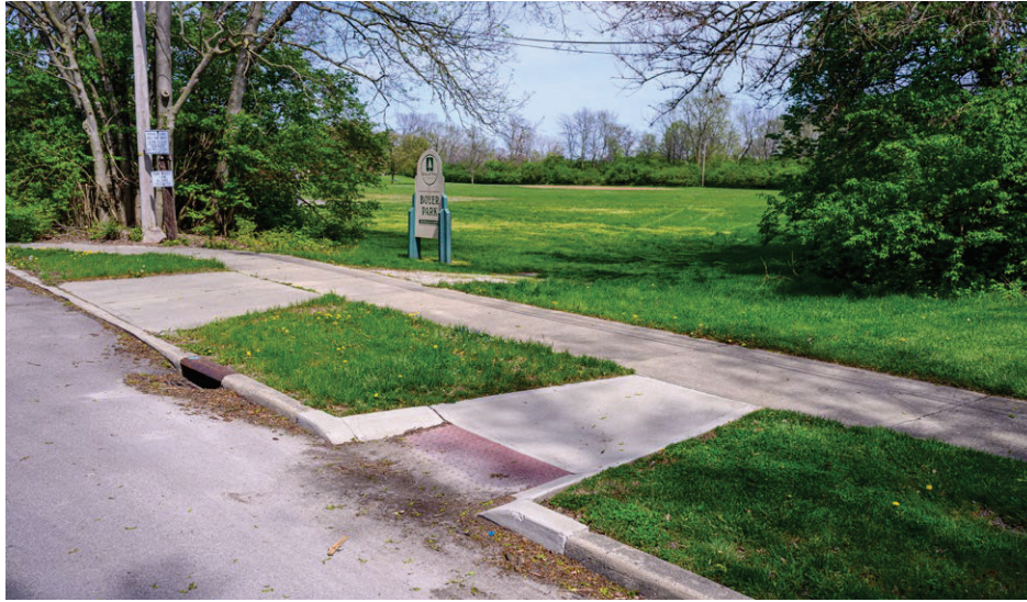
Parking bumpers at Joe Reardon Skate Park are too close together for a wheelchair user to roll between them onto the adjacent path.
