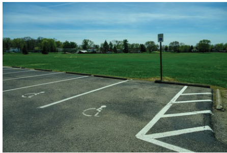
Accessible parking stalls at Community Park need to be cleared of grass with access aisles painted and at least one stall made into a van-accessible space with a sign.
