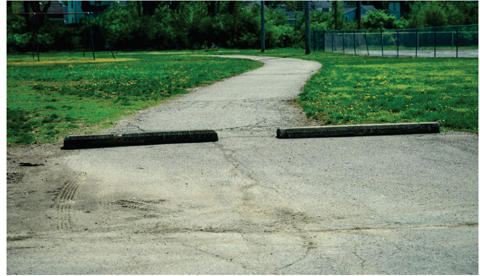
Spots labeled with the accessibility symbol at Treasure Island Park are not ADA-compliant because they should be paved.
