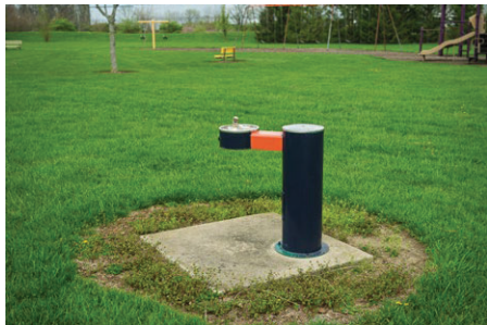
A water fountain at Carriage Crossing Park can be rolled under by a wheelchair user, but is disconnected from pavement connections.
