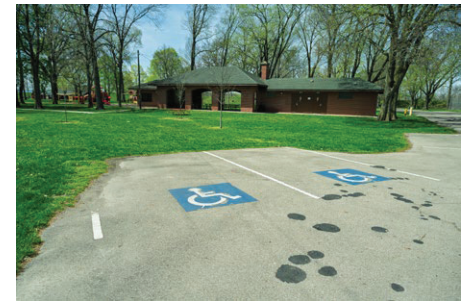
Accessible stalls at Duke Park that do not have a striped aisle to access each space, and the current aisle is not wide enough.
