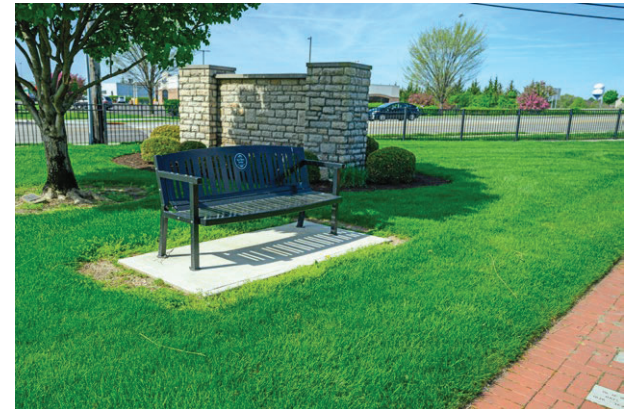
The bench at Mayor's Park is accessible and needs a paved connection to the nearby paver walkway.
